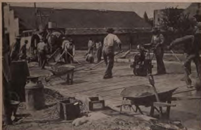
Laying Vibrolithic Pavement.
